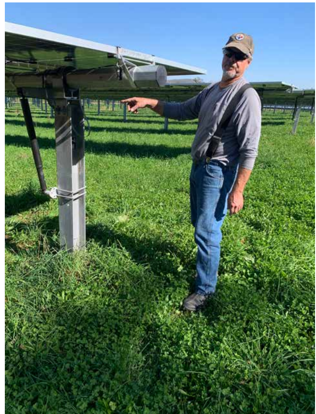
Solar panels used with sheep grazing are nearly six feet high, higher than low-rack panels. Photo by Tom Daniels.
