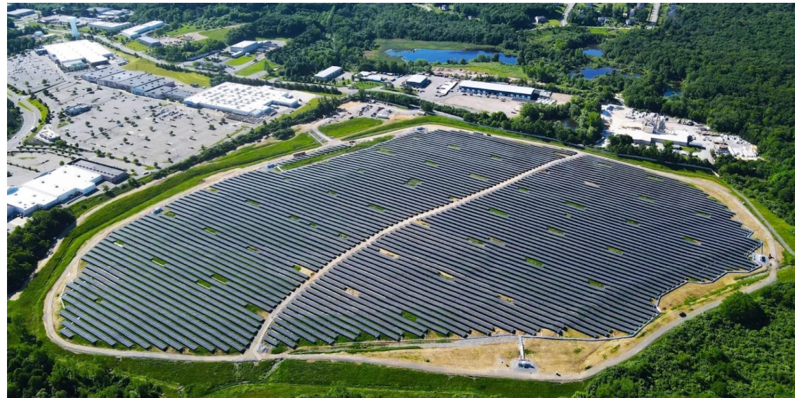
The largest landfill solar project in North America, a 25.6 megawatt (MW) solar farm in Mount Olive, New Jersey
