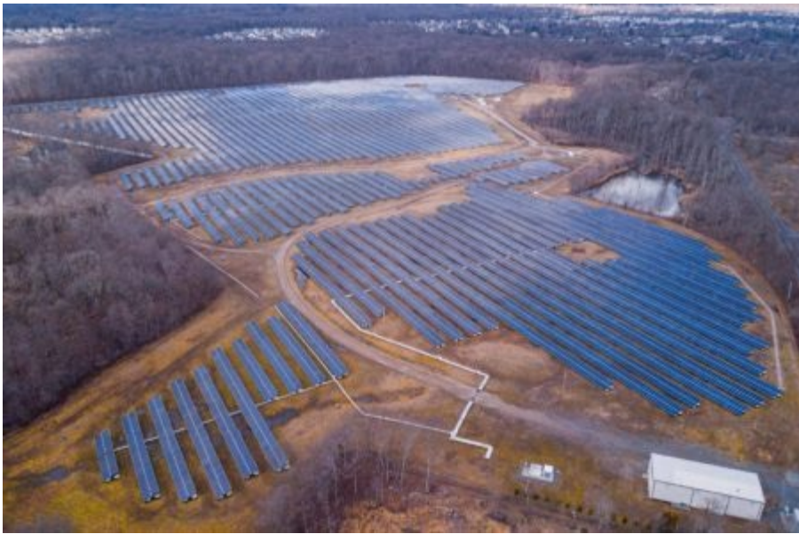
The 13-megawatt New Road Solar Project, constructed on a landfill site in New Jersey
