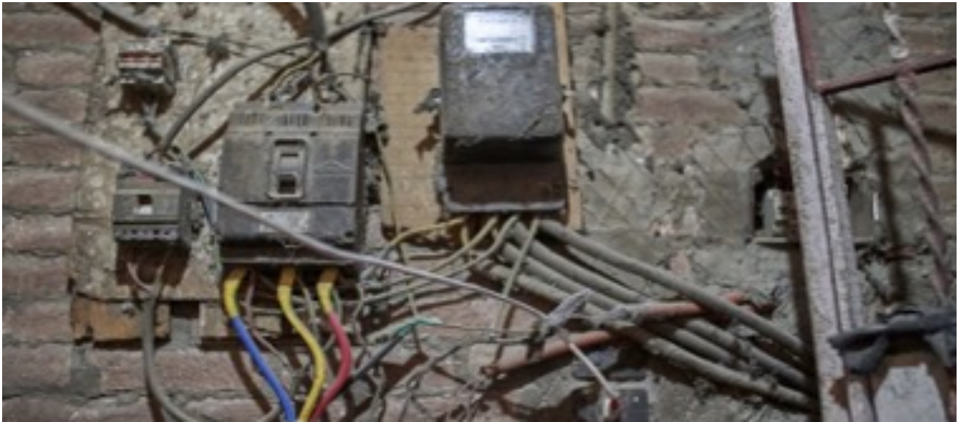
FIGURE 9: ILLEGAL CONNECTIONS—SEVERAL CABLES CONNECTING TO ONE METER
