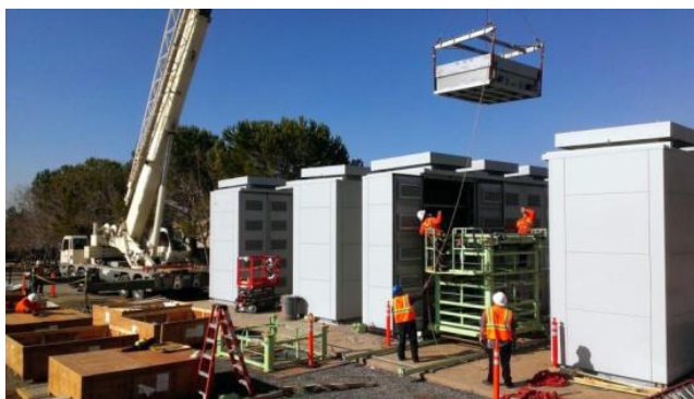
Figure 2: Installation of PG&E's Yerba Buena battery system (Pacific Gas and Electric Company 2015)
