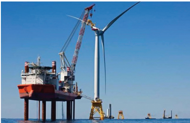
FIGURE 5: HEAVY-LIFT JACK-UP VESSEL IN OPERATION
