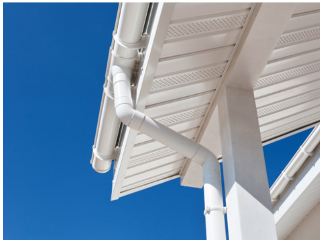
FIGURE 3: NEW RAIN GUTTER
