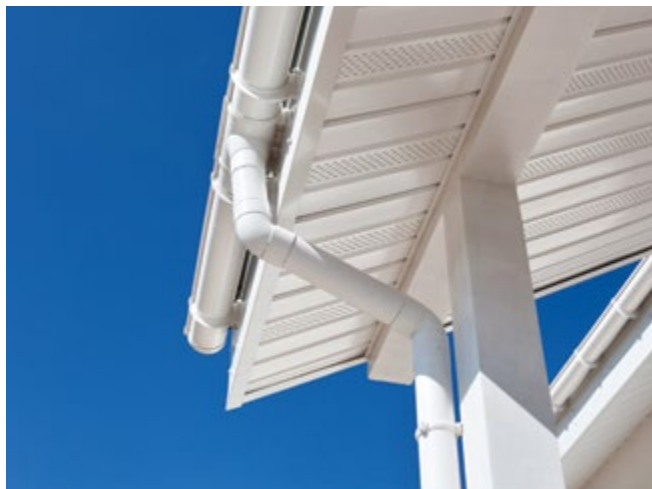
FIGURE 3: NEW RAIN GUTTER
